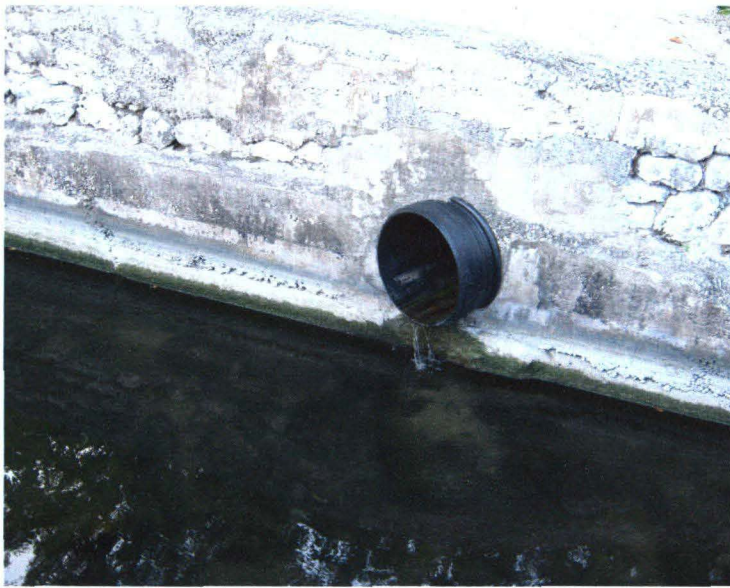
Stormwater inlet into canal, south of HWY 7
