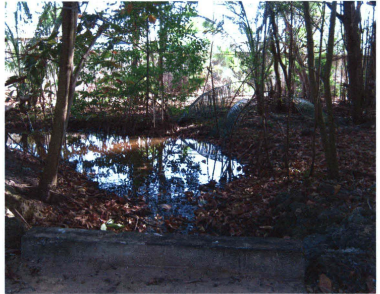
Storwater Ditch in southwest corner of Sancturay, looking south
