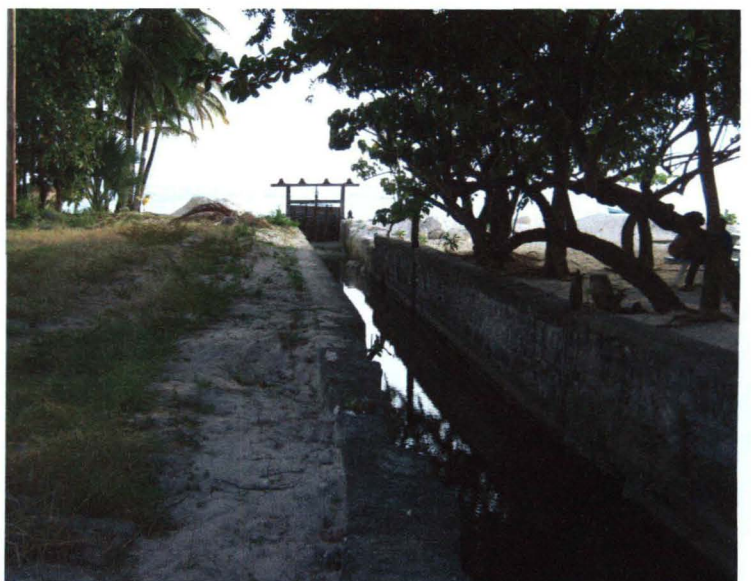
Canal and sluice gate south of HWY 7, looking south
