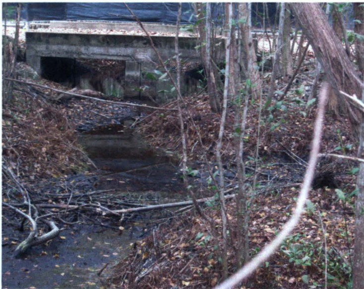
Stormwater inlet from west to Sanctuary's west Stormwater Ditches
