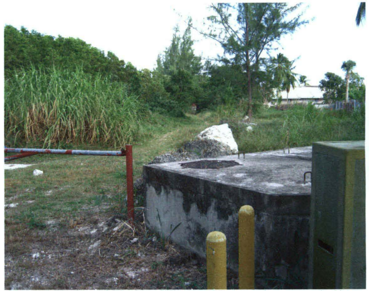
Access Road to Sewage Treatment Plant and lift station for sewage, looking east
