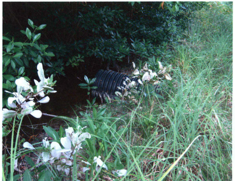
West end of culvert from freshwater marsh into Bisecting Canal
