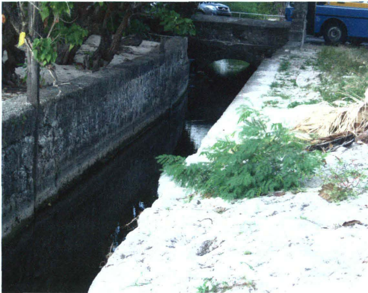
Canal, looking north towards HWY 7.
