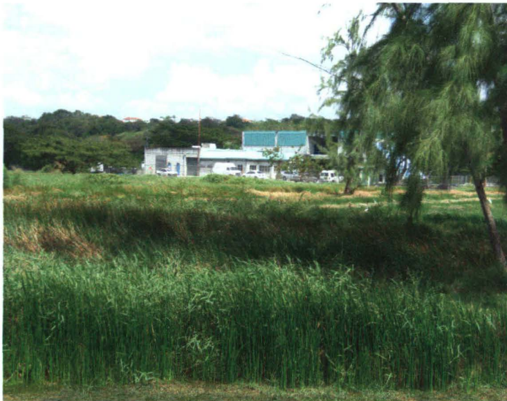
Sewage Treatment Plant, looking north
